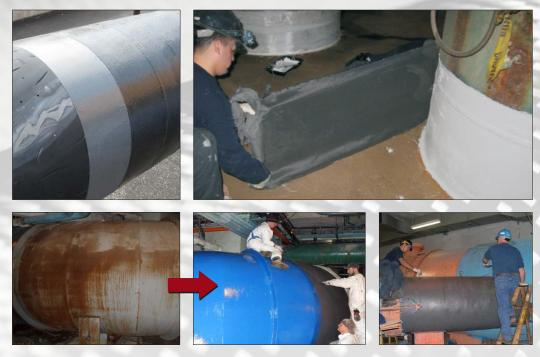
*METALCLAD*<sup>®</sup> *DuraWrap*<sup>®</sup> can be applied to the interior and / or exterior of piping and equipment to both seal and strengthen these components. When applied to the interior walls of underground or otherwise inaccessible piping, *METALCLAD*<sup>®</sup> *DuraWrap*<sup>®</sup> can effectively repair and restore piping integrity without expensive excavation and replacement.
